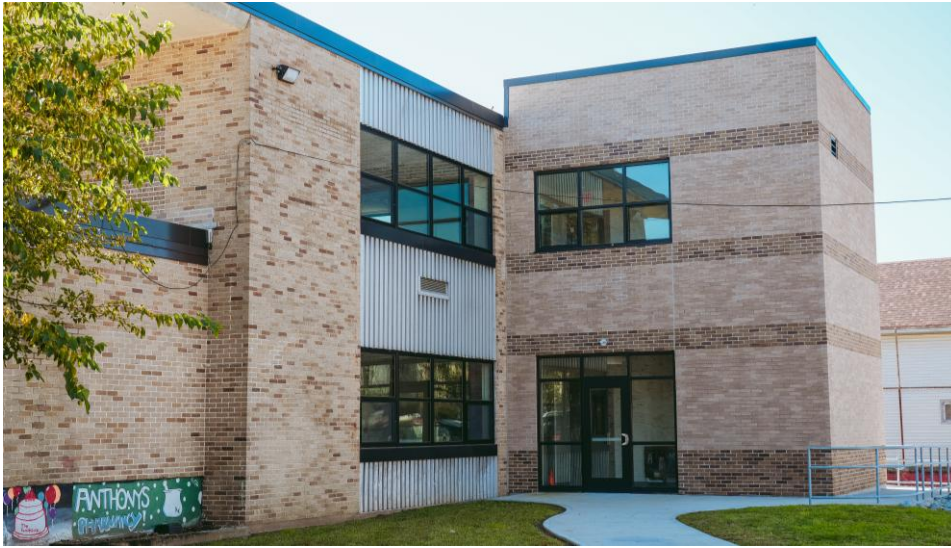
▲ Exterior of the existing building
