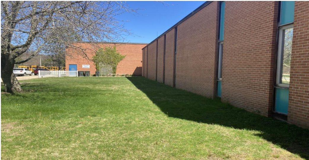
▲ Exterior of the existing building
