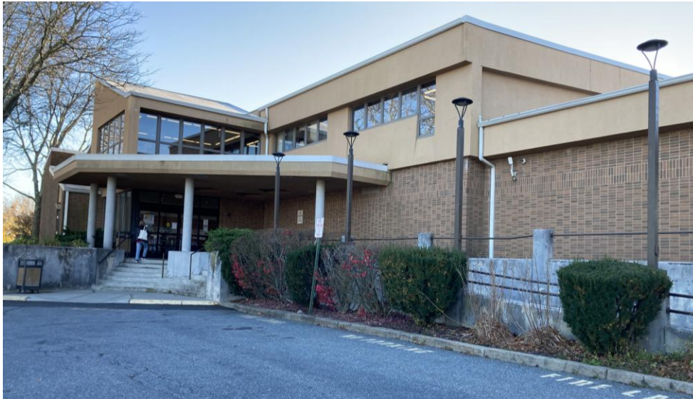
▲ Exterior of the existing building
