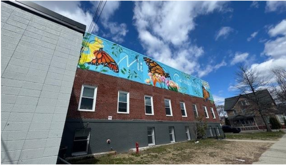
▲ Exterior of the existing building
