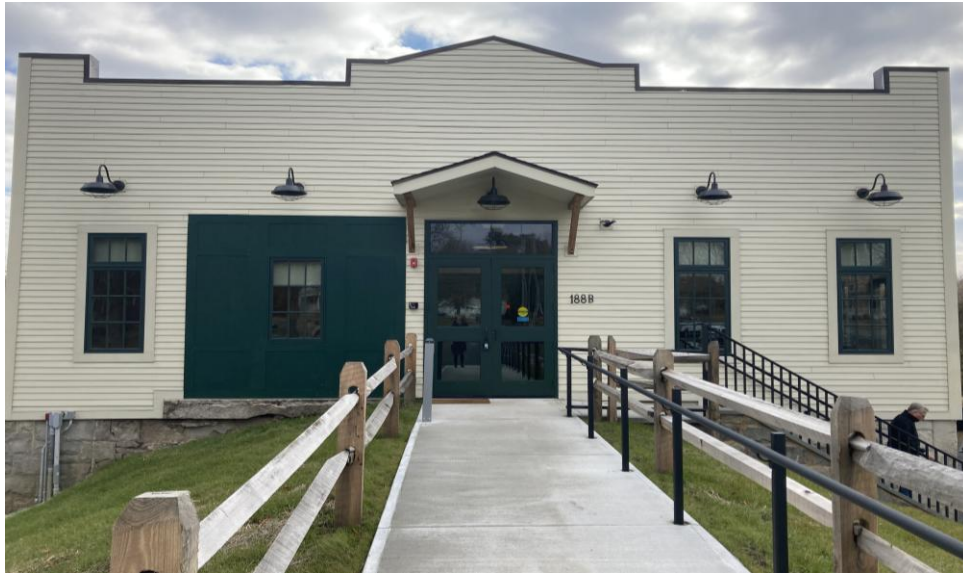
▲ Exterior of the existing building post renovation
