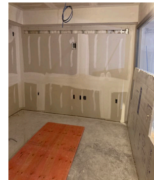
▼ Interior repairs continue with drywall installation throughout.
