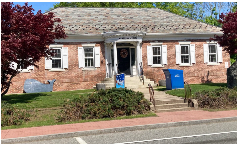
▲ Exterior of the existing building from Putnam Pike
