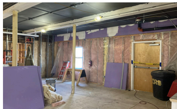
▼ Garage bay conversion continues
