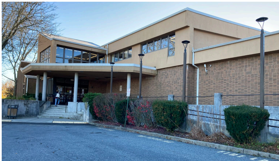
▲ Exterior of the existing building
