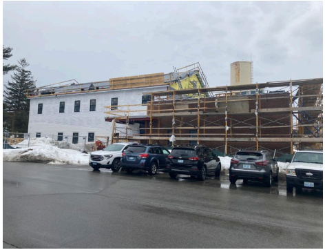
▼ Exterior brick veneer complete
