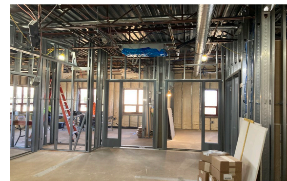
▼ Framing and rough-in occurring throughout
