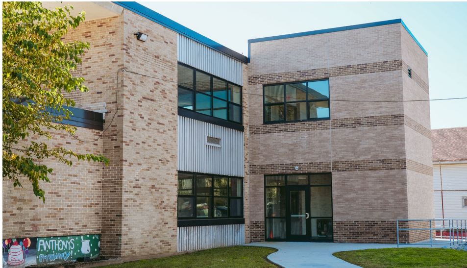
▲ Exterior of the existing building
