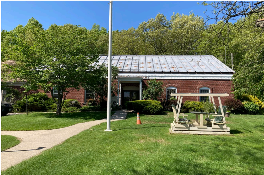
▲ Exterior of the existing building from parking lot
