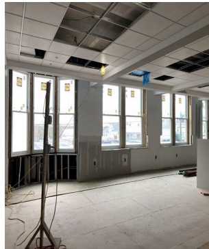
▼ Interior repairs continue with drywall installation throughout.
