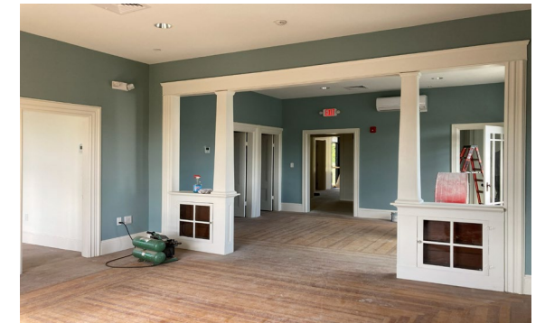
▼ Interior finish work completed
