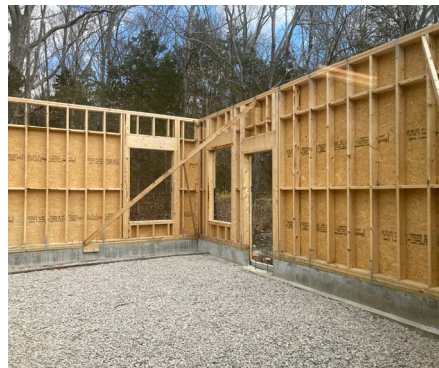
▼ Walls of the rear addition are being erected.
