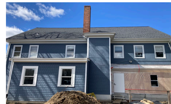
▼ Rear addition has been erected and vinyl sided.
