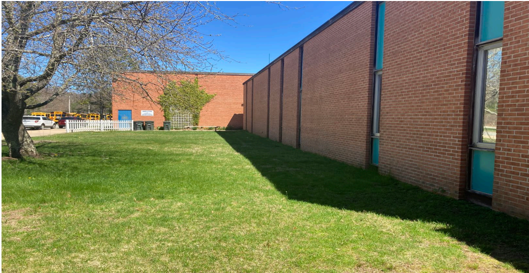
▲ Exterior of the existing building
