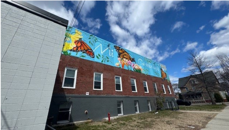
▲ Exterior of the existing building
