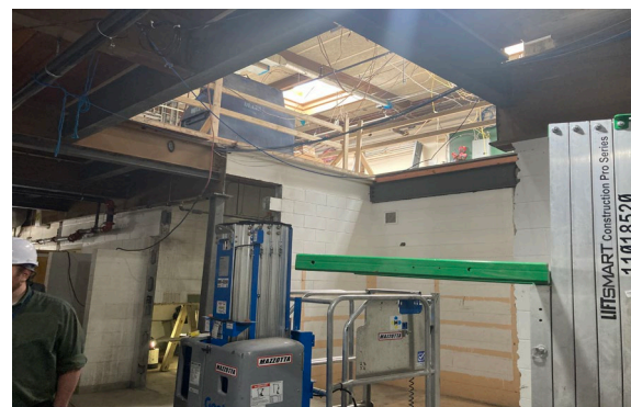
▼ Cut out for the new central staircase
