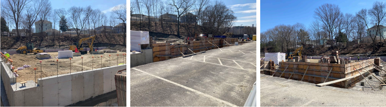
▼ Foundation work for the new multipurpose center ongoing.
