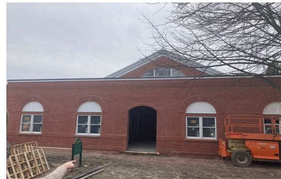
▼ Exterior masonry & windows are complete
