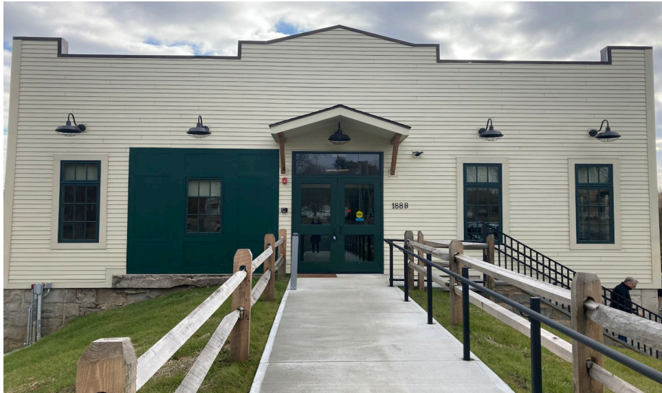
▲ Exterior of the existing building post renovation
