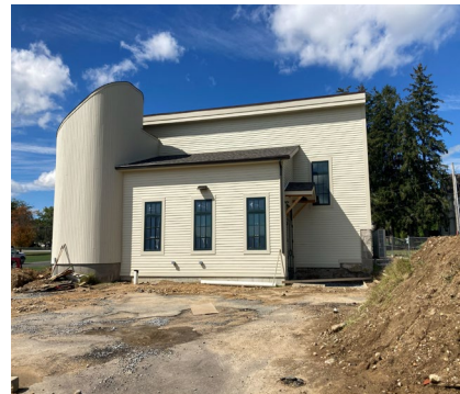
▼ Rear exterior mid-renovation
