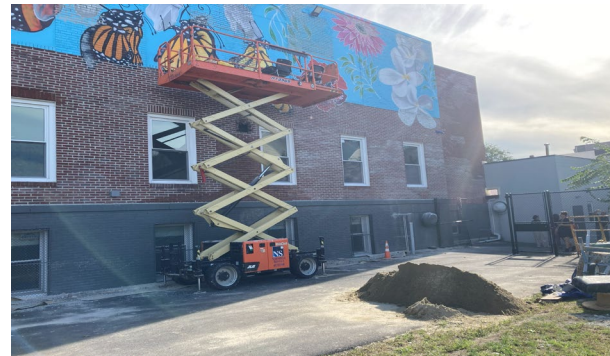
▼ Exterior brick repointing nearly complete
