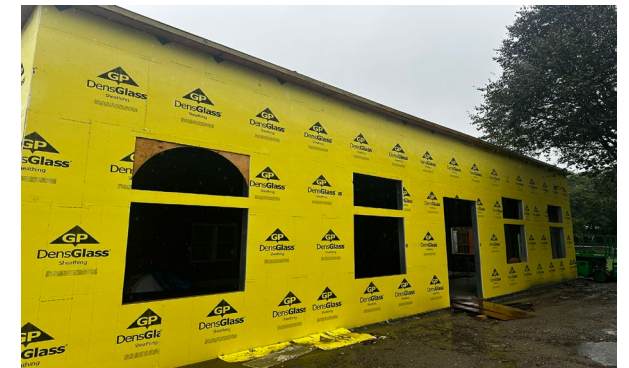
▼ Waterproofing exterior is underway
