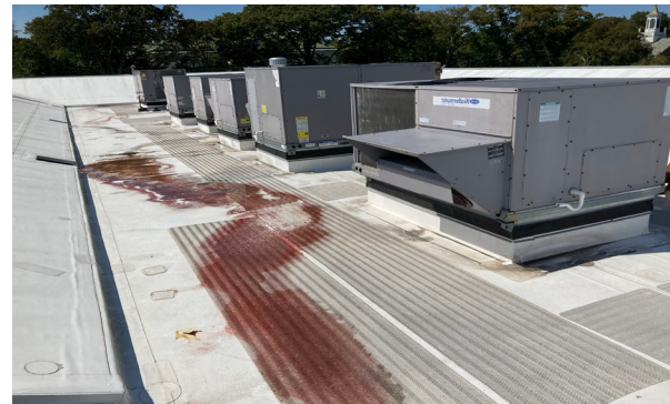
▼ Roof view – building wide system upgrades
