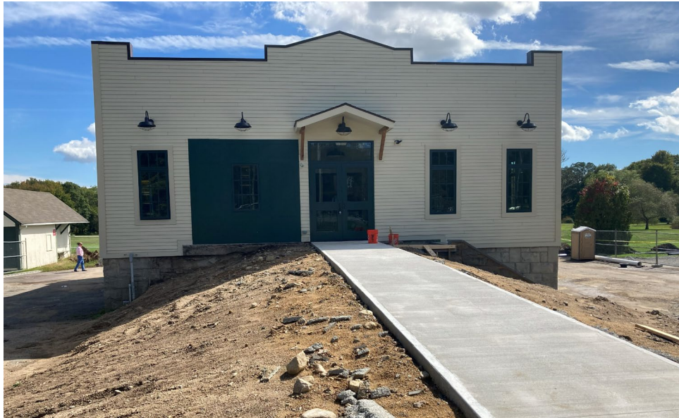
▲ Exterior of the existing building mid renovation
