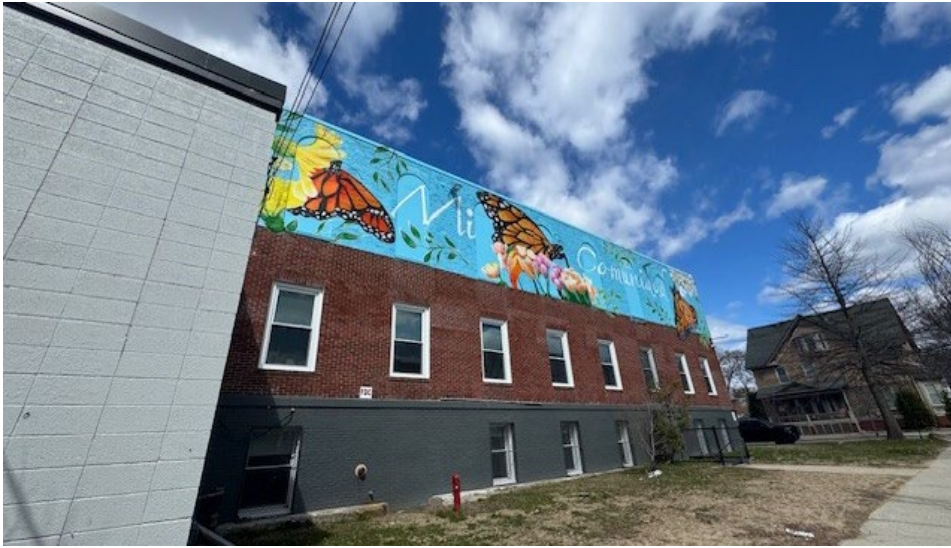
▲ Exterior of the existing building
