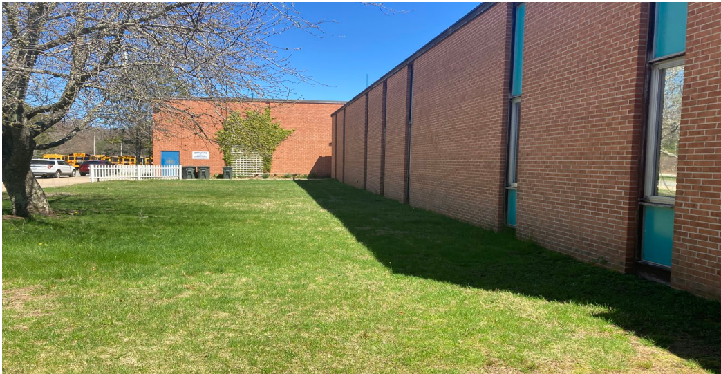
▲ Exterior of the existing building
