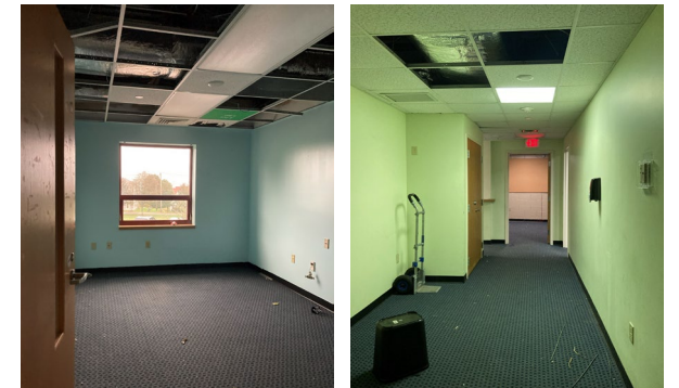
▼ Gallagher wing emptied for gut renovation
