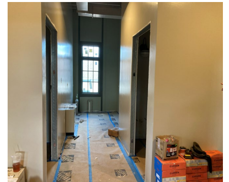
▼ Build out of rooms underway
