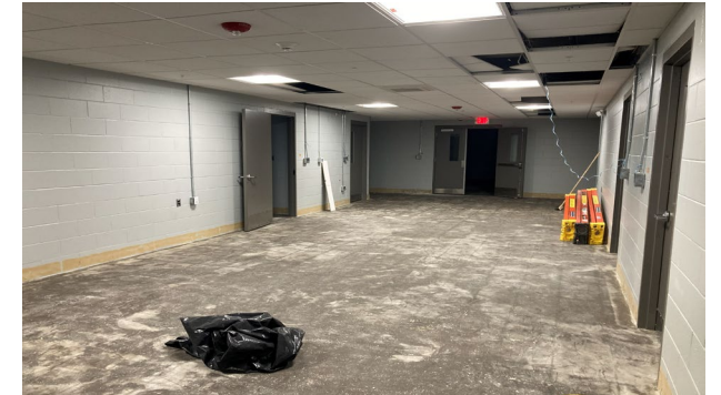
▼ Basement level ready for new flooring
