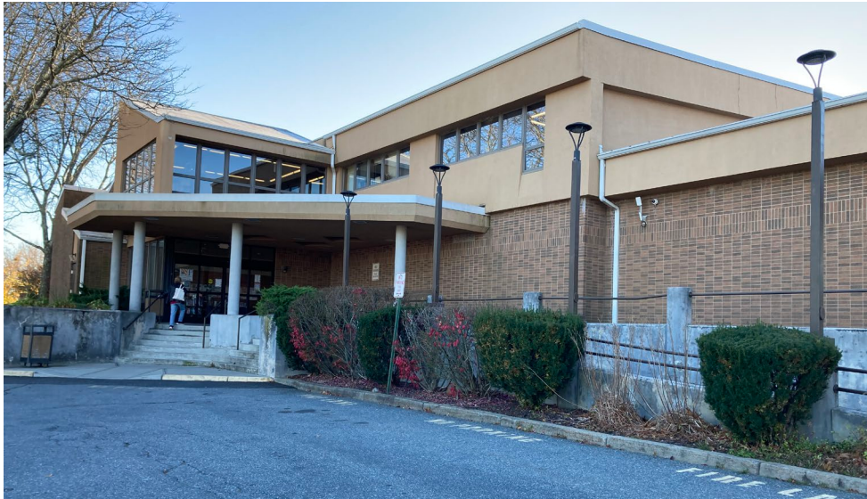
▲ Exterior of the existing building
