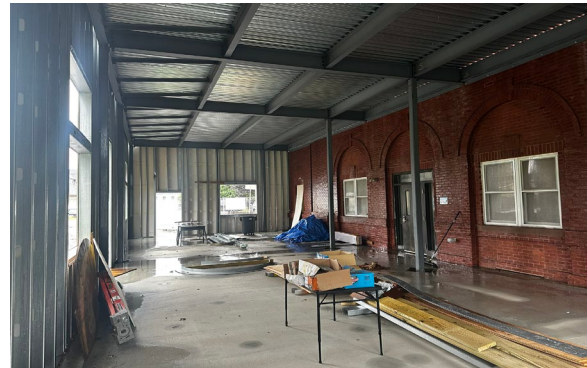
▼ Structural steel erected
