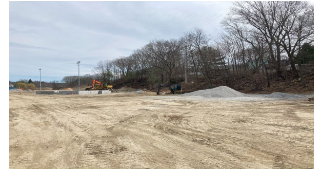
▼ Site work complete
