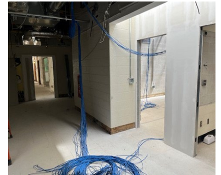
▼ Wiring work continues
