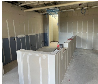
▼ Drywall is underway
