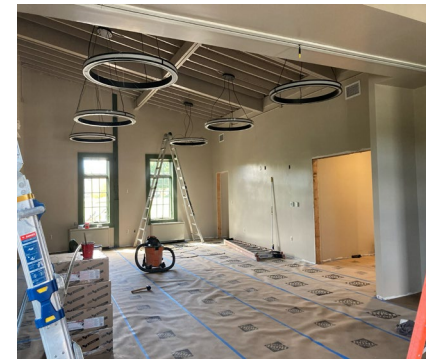
▼ Overhead fixtures installed
