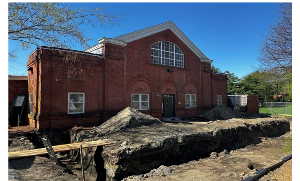
▼ Sitework completed for foundation pour
